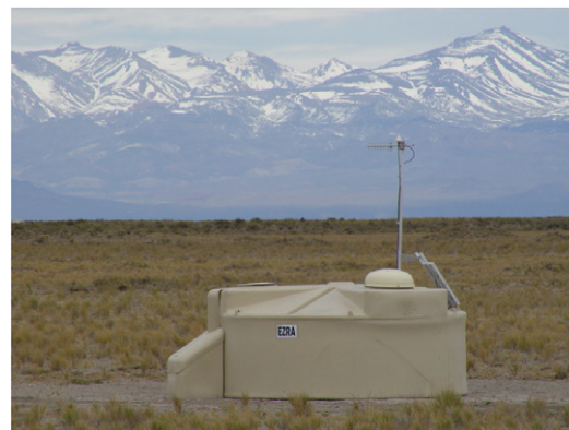
Figure 2. One of the surface detectors of the Pierre Auger Observatory. The detector is filled with 12 tonnes of pure water. In the figure one can see the battery box at the left bottom of the detector, a solar panel and an antenna. It is also possible to see a dome on top which covers the electronics of the detector. The detector is fully autonomous and has no wire connection to the central data acquisition system.
